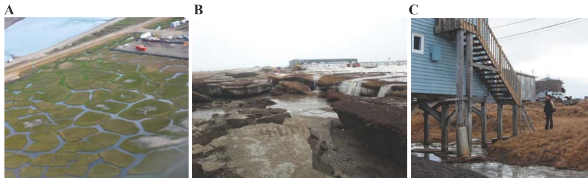
Figure 7. A. Ecosystem changes related to roadside impoundment of water (Photo: D.A. Walker); B. Damage to the built environment. Northern end of the Dalton Highway looking south near the Deadhorse Airport during height of a flood May 19, 2015, showing an area of thermokarst collapse. (Photo: Alaska DOT & PF). C. New Point Lay house with foundation that is threatened by thermokarst. Note subsidence and ponding in a newly developed ice-wedge polygon trough around the pilings supporting the house; the bottom of the steps leading to the second story used be at the ground surface (Photo B. Grunau).
