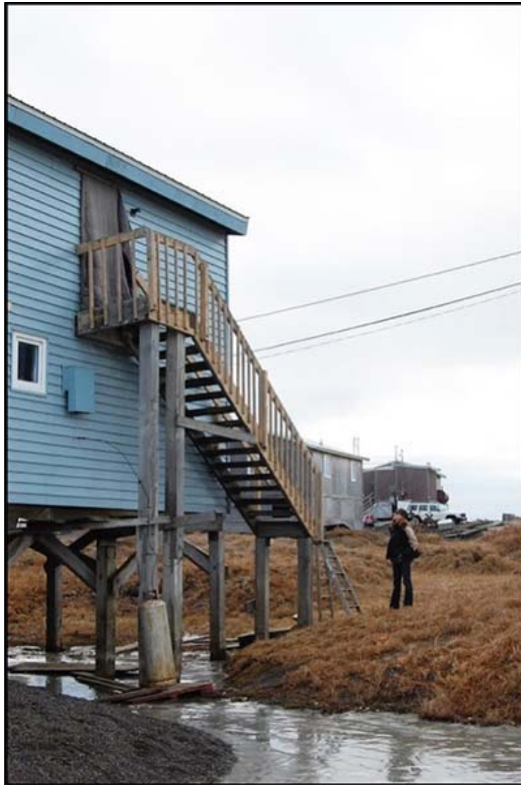
Figure 4. Subsiding ground beneath Point Lay house. In late 1980s, the base of the steps was at ground level and there was no thermokarst. Photo: Courtesy of CCHRC.
