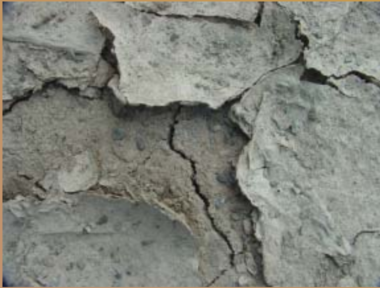
Mould Bay, Desiccation cracks.
