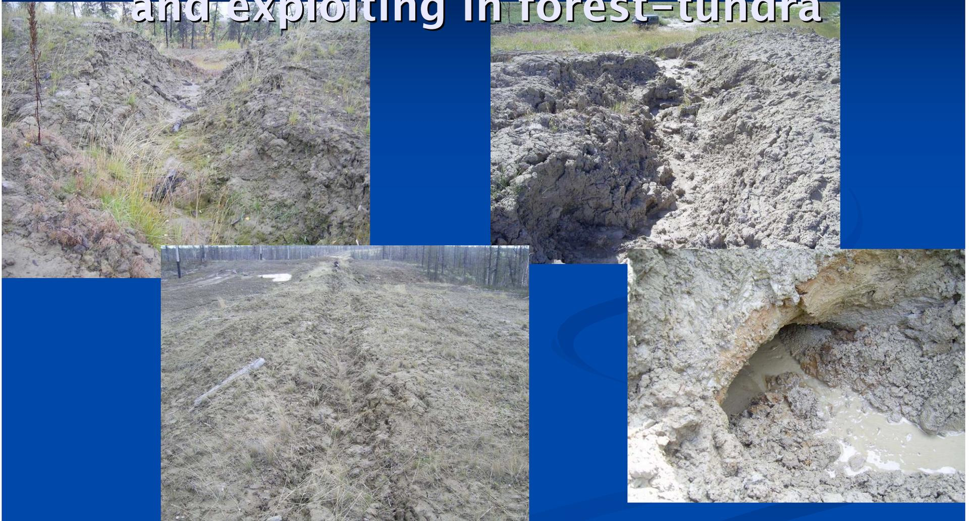
Even in discontinuous permafrost cryogenic processes are activated immensely on the construction sites. In continuous permafrost in tundra, with massive ground ice consequences will be much stronger
