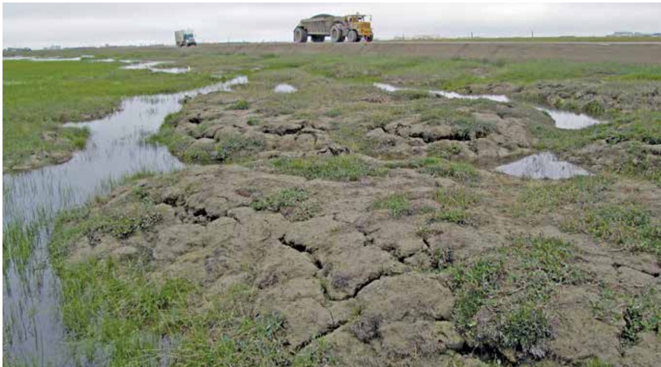
Figure 2.14. Thermokarst and eroded high-centered polygons that have developed in a flooded area between the road and the margin of a drained lake basin. Photo: IMG_0783.
