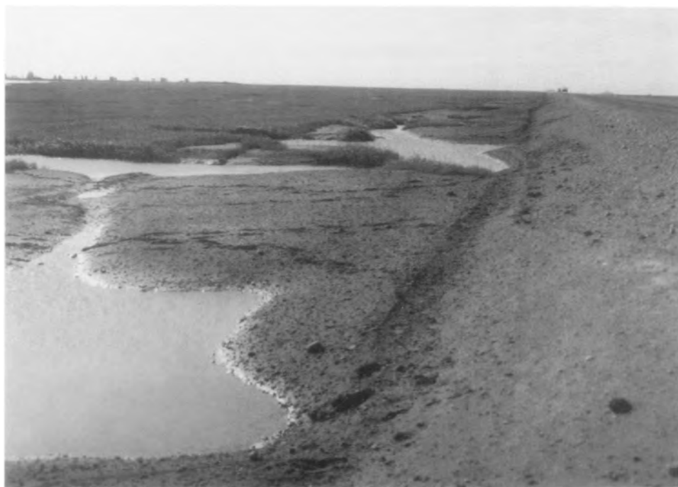
FIGURE 6. Roadside area along the Prudhoe Bay Spine Road. Within 10 m of the road vegetation has been buried by road dust. Impoundments are thermokarst features that form along eroded ice wedges.
