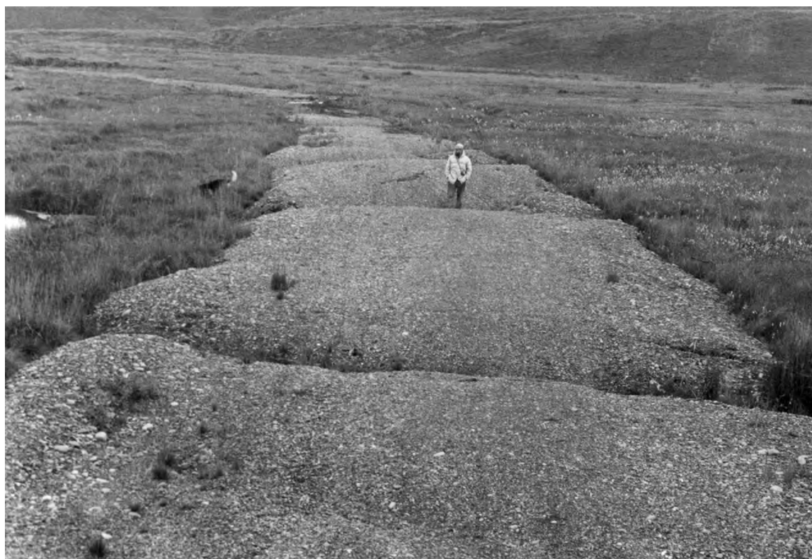
FIGURE 6-4 Roadway destroyed by thawing ice edges near Umiat. Gravel fill was not thick enough to replace insulating effect of the organic mat, which it destroyed. Photograph by Gordon Greene. SOURCE: Lachenbruch 1966.
