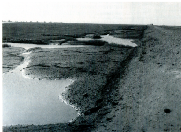
Figure 2. Roadside area along the Prudhoe Bay Spine Road. Within 10 m of the road vegetation has been buried by road dust. Water collected in the ice-wedge troughs is actively eroding the centers of some polygons and converting previous low-centered polygons to high-centered polygons. Photo is a 1983 road transect that would be resampled for this project (Walker and Everett, 1987). Thermokarst has spread much more widely in the 25 years since this photo was taken.
