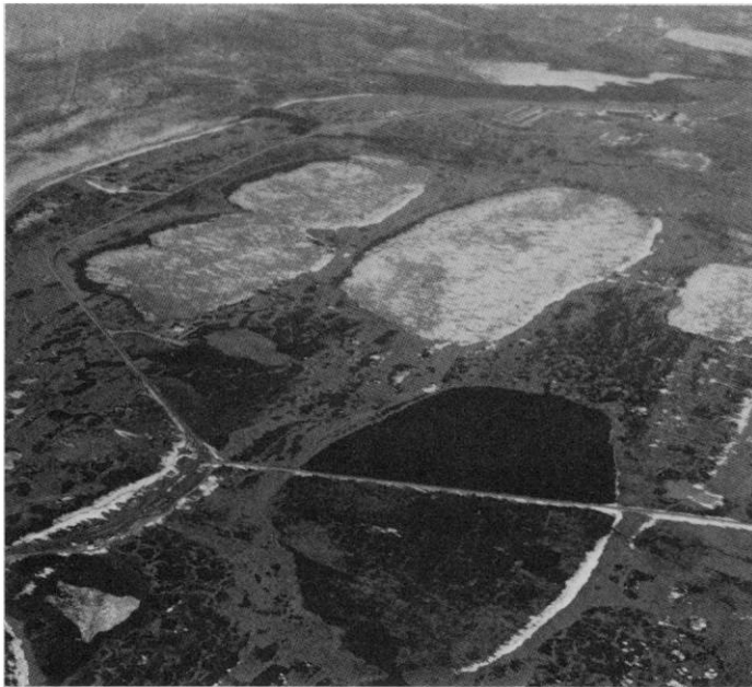
Fig. 2. A large drained lake basin that was traversed by a road in the Prudhoe Bay Oil Field. The area farthest from the camera was flooded to about 1 to 1.5 m in depth. The foreground area is not flooded and contains many sites suitable for waterfowl nesting. Note the numerous ice-covered thaw lakes and the ice-free runoff water in the flooded lake basin. Numerous other roadside impoundments are visible along the road leading into the background. [Photo by L. Klinger, 21 June 1982]
