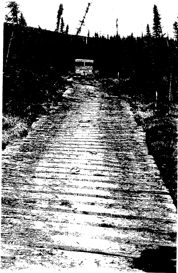
Figure 4. ORV trail in taiga woodland, with surface protected by native timber "corduroy" and by sawn timber puncheon.
