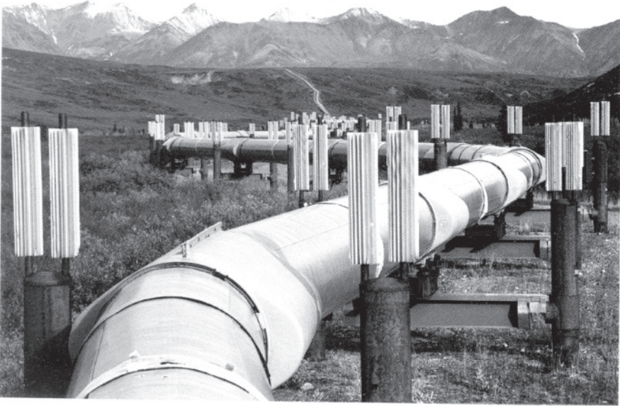
Figure 1.7 A forest of refrigerated pilings supports the trans-Alaska pipeline where it snakes through the Alaska Range north of Isabel Pass. See also Plate 2.
